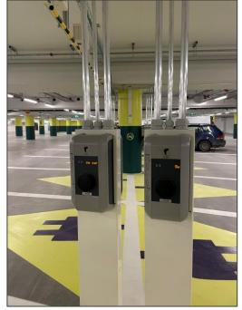
*Figure 12. Installed EV chargers in Lippulaiva parking garage. Source: authors.*
