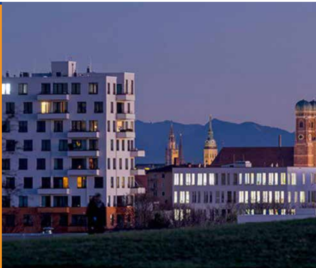
Figure 10 : Overview of Munich from the Ackermannbogen, a residential energy efficient development.
